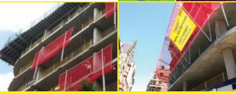
SAFETY NET SERVICES HAVE DEVELOPED A UNIQUE SYSTEM FOR RAISING & FITTING SAFETY NET FANS WITHOUT THE NEED TO RELY ON THE USE OF A TOWER CRANE. THIS ENSURES THE FANS ARE INSTALLED IN A SAFE AND EFFICIENT MANNER WITH MINIMUM DISRUPTION TO OTHER TRADES. **1**
